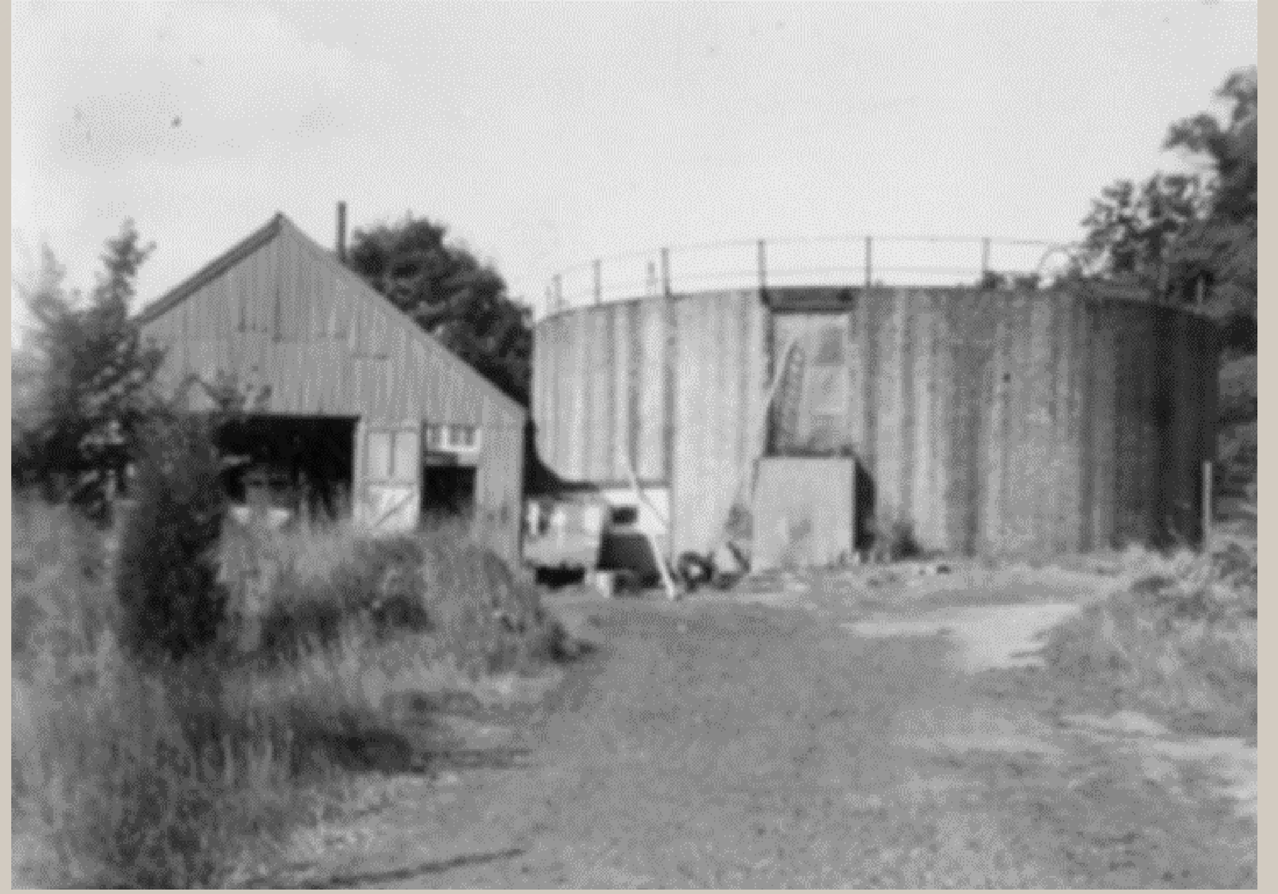
Lower diesel storage tank c. 1950
