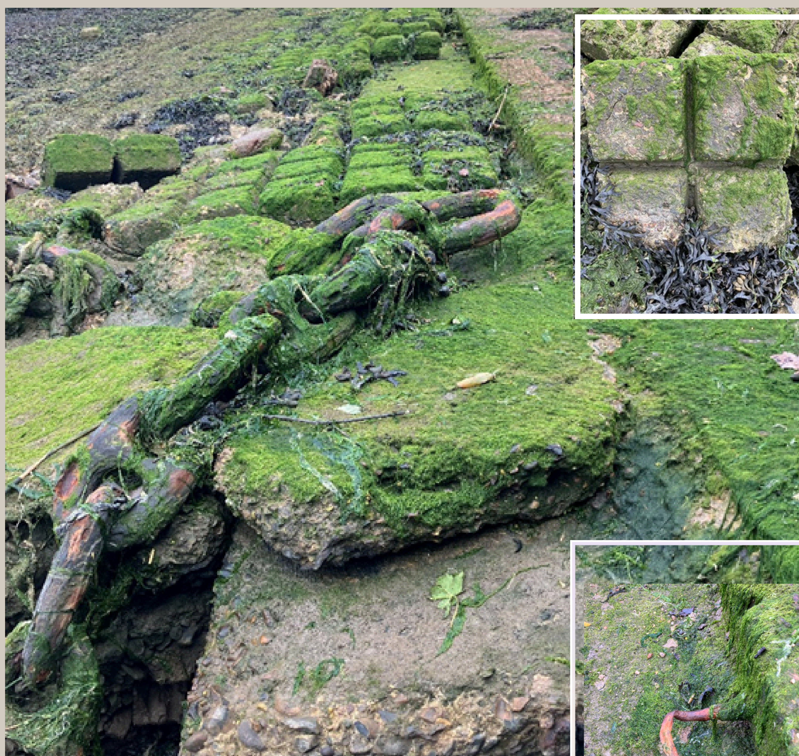
Some remains of the metal hooks to secure this can still be seen.
