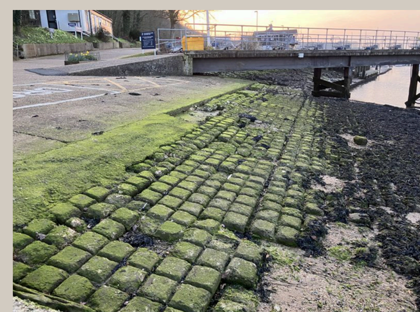
11. Flexible matting – chocolate blocks - in the intertidal zone. Much of the matting has disappeared as it no longer reaches to low tide. The matting was mostly laid in 15 block sections, 3 x 5. 62 cm (24 in) x 102 cm (40in). The mats are 12.7 cm (5 in) thick. Each block is of a similar design of moulded concrete.
